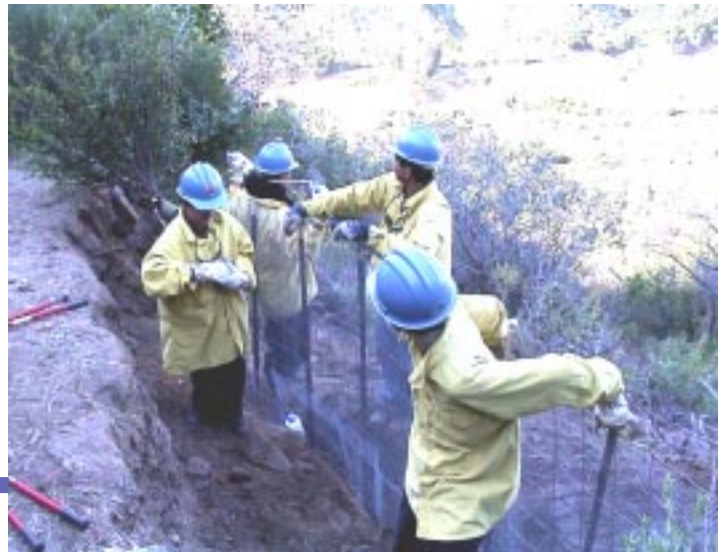
Installing mesh wall screen along blown out sections of Oak Springs
