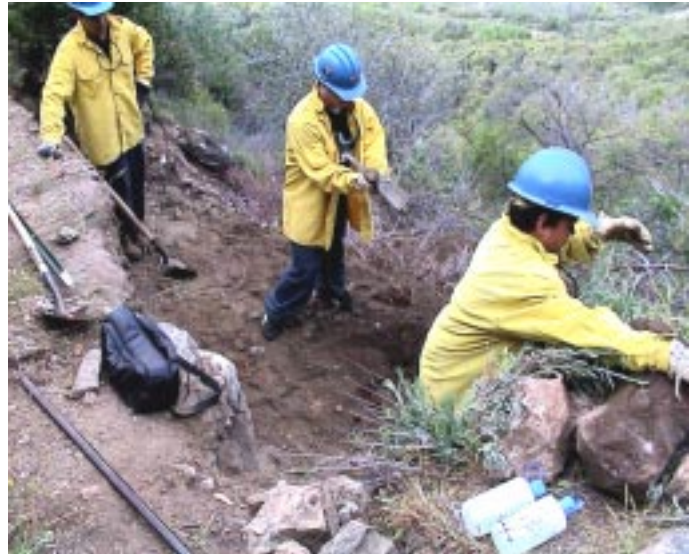
Installing mesh wall screen along blown out sections of Oak Springs
