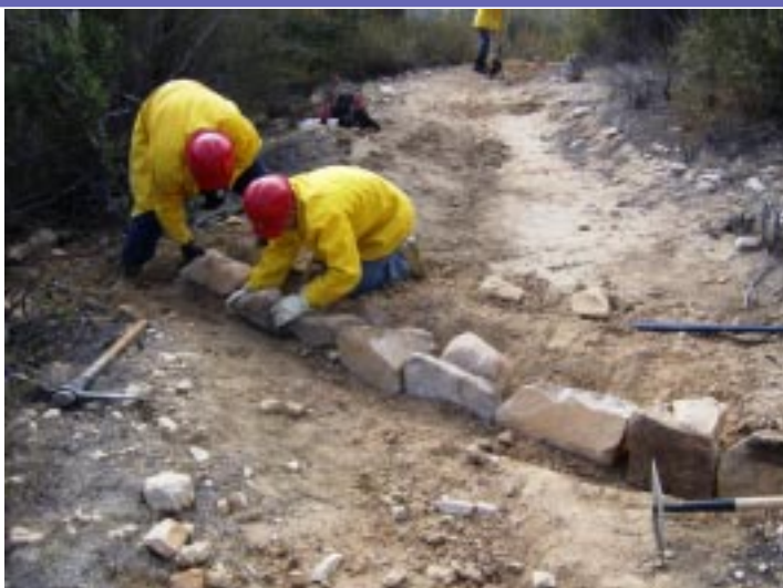
William S Hart UHSD Students Installing a Water Bar
